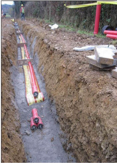
Plate 4-8 Typical Cable Trench View
