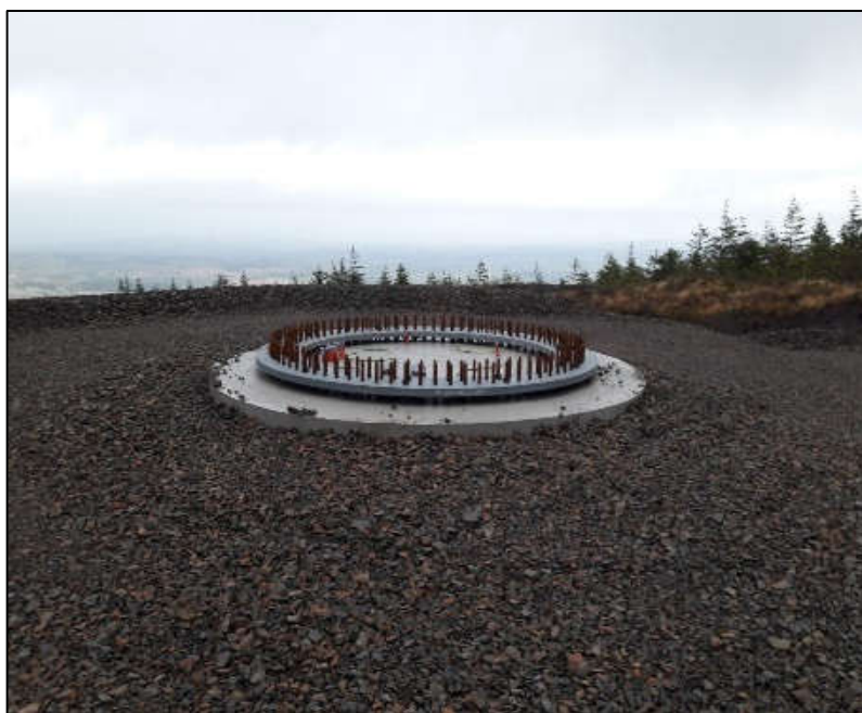
Plate 4-3 Finished Turbine Foundation
